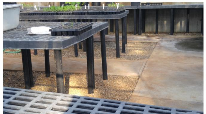
FIGURE 4. A small greenhouse with concrete walkways and gravel under the benches to support drainage.
