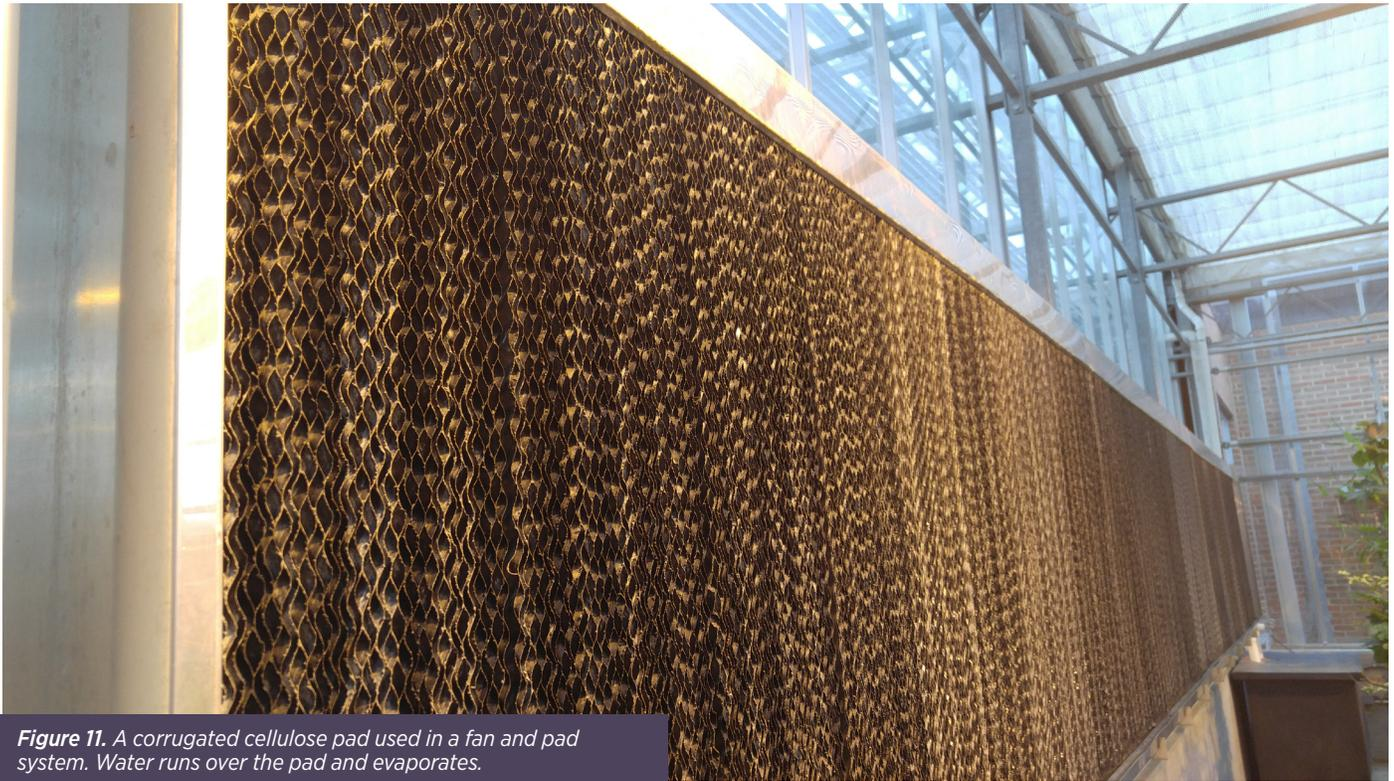
*Figure 11. A corrugated cellulose pad used in a fan and pad system. Water runs over the pad and evaporates.*
