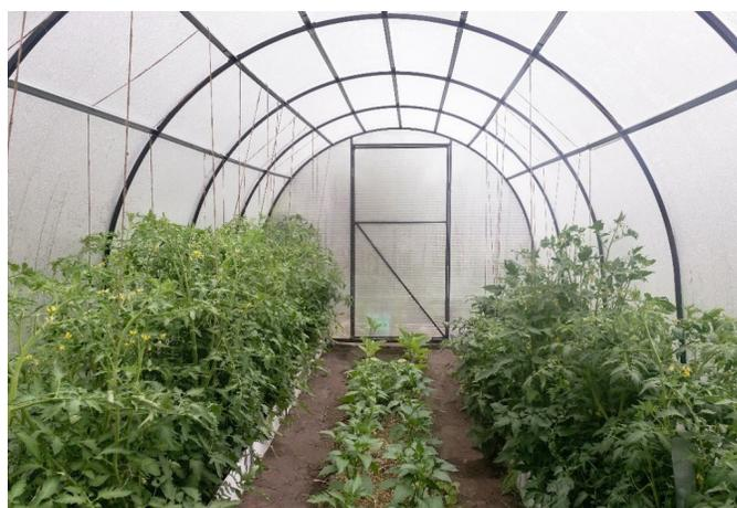
**FIGURE 1.** This is the inside of a hoop (or Quonset) style structure with polycarbonate covering. While this design would work well in the spring and fall seasons, the doors are the main method of ventilation and there are no heaters or cooling pads. Since this structure is more a high tunnel than a greenhouse, there would be limits to the growing season in this structure. Image: Shutterstock
