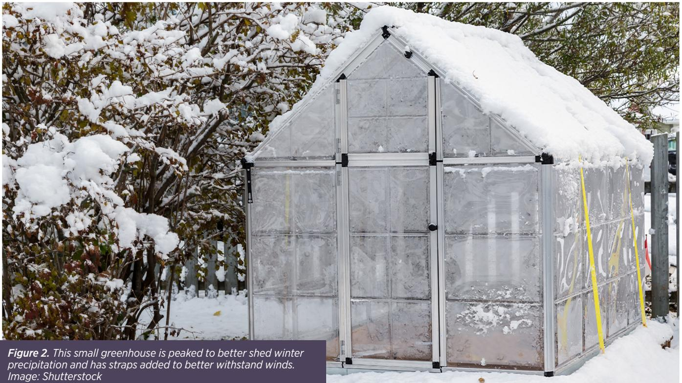
**Figure 2.** This small greenhouse is peaked to better shed winter precipitation and has straps added to better withstand winds.
