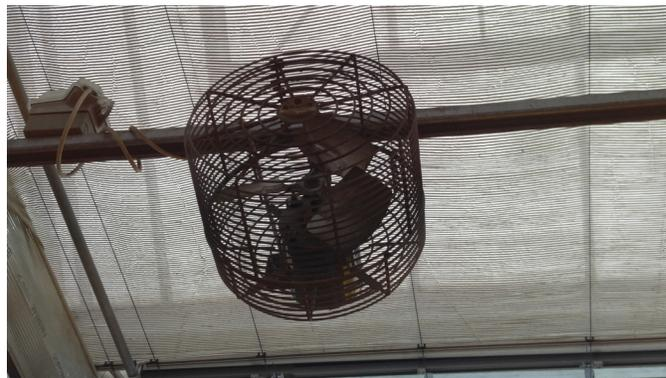
*Figure 8. A circulation fan that can be used to mix warm and cool air and maintain even humidity throughout the greenhouse.*
