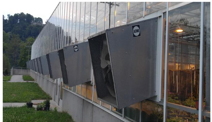
*Figure 10. Evaporative cooling is accomplished as an exhaust fan pulls air out of the greenhouse and pulls air through a pad on the other side of the greenhouse. These fans are available in many sizes to fit a range of greenhouse structures.*
