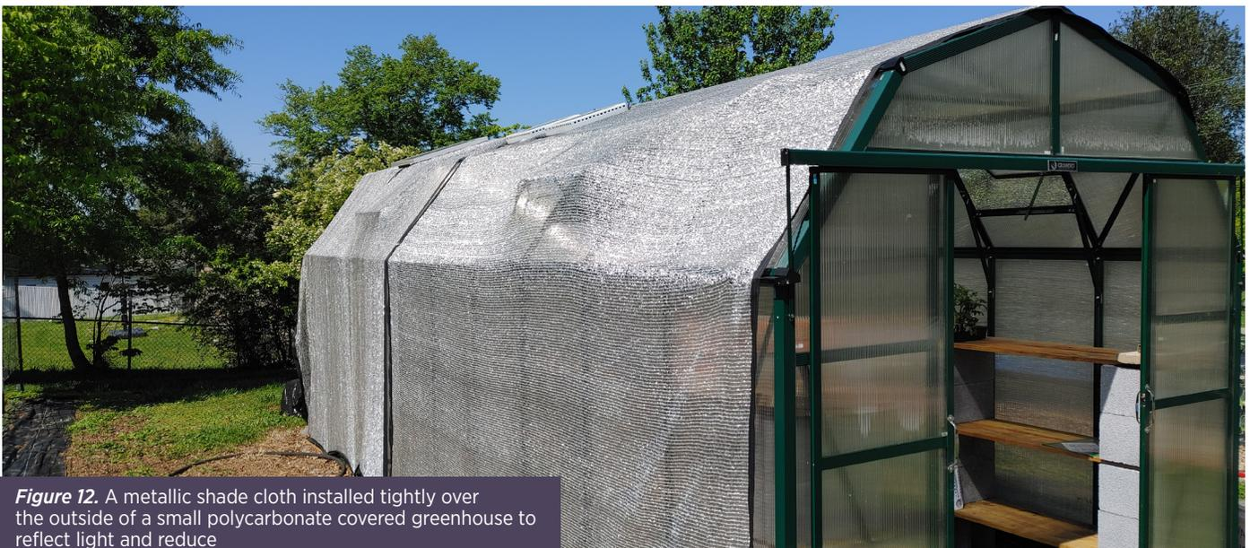
*Figure 12. A metallic shade cloth installed tightly over the outside of a small polycarbonate covered greenhouse to reflect light and reduce*
