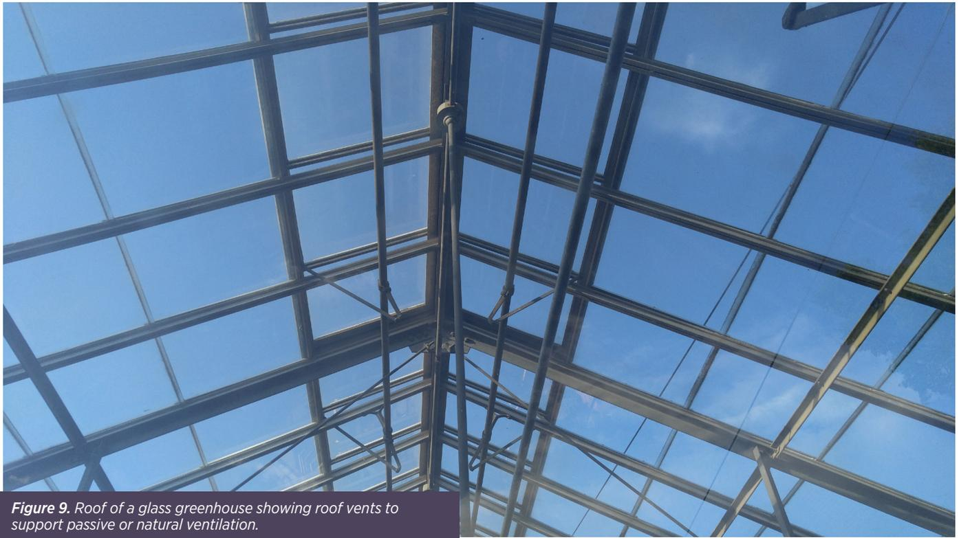
*Figure 9. Roof of a glass greenhouse showing roof vents to support passive or natural ventilation.*
