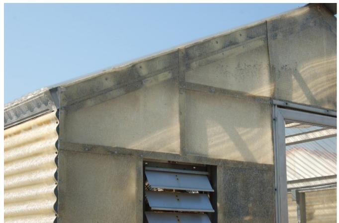
*Figure 7. Fiberglass reinforced plastic greenhouse material that has degraded in a way that greatly reduces light transmission.*
