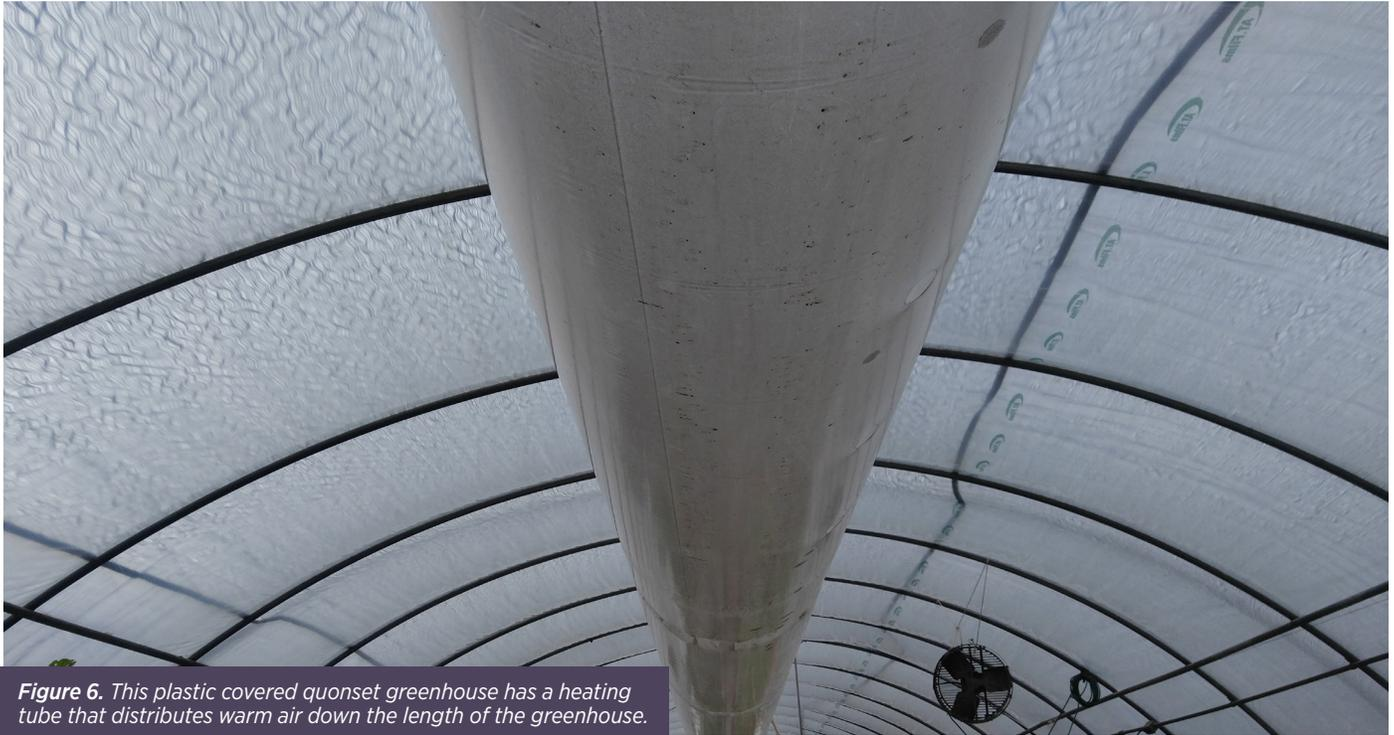
*Figure 6. This plastic covered quonset greenhouse has a heating tube that distributes warm air down the length of the greenhouse.*
