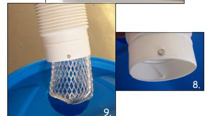
\*Note: The sump pump hose kit comes with a 24' foot corrugated hose, 2 different size adaptors and 1 hose clamp. These directions use the 1 1/2" adaptor, 1/2 of the hose, and the hose clamp. To make a 2nd rain barrel using the 1 1/4" adaptor included in the kit, you will need the following supplies: 1 steel hose clamp; 1 (1 1/4") steel conduit locknut; 1 (1 1/4") Schedule 40, 90° elbow; and a 1 5/8" hole saw.
